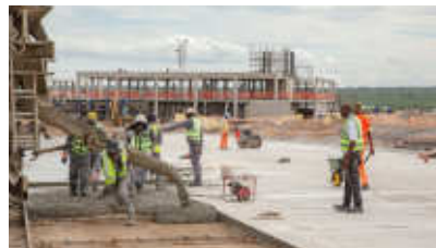
There are around 1,160 people on site with more than 570 labourers from the local area.
